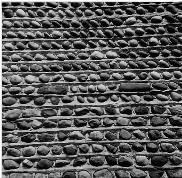
Lake-washed cobblestones on top half of the picture and field cobblestones on bottom half. Also, note the anchoring stones in the center of the picture. The Charles Hoagland house in Williamson Township.
